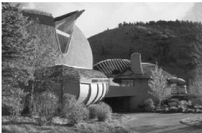
Bart Prince: Whiting-ház Sun Valley, Idaho, USA, 1989-1991
